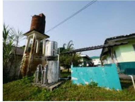
school water tank
